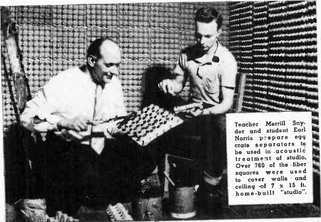
Teacher Merrill Snyder and student Earl Norris prepare egg crate separators to be used in acoustic treatment of studio. Over 760 of the fiber squares were used to cover walls and ceiling of 7 x 15 ft. home-built "studio".
