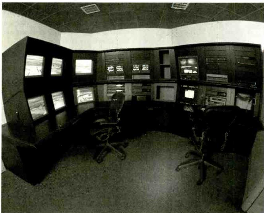
Pictured here is the fully integrated audio/visual control system for recording/playback, remote viewing, and coordinated communication of a simulation in progress. Equipment includes six RGB monitors, five video monitors (one for quad-split viewing), six VCRs (one Betacam and five VHS), one DVD player, one multi-disc player (laser/CD), timecode units, video text generator, patch bays, microphone, and Crestron touch panel system control.
