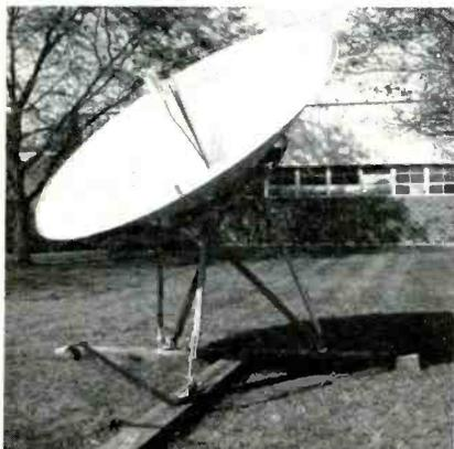
Combination packages of 10-foot and 12-foot antennas and 120° and 100° LNAs are available.
