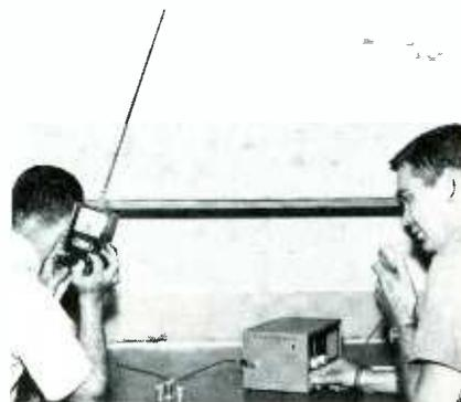
Fig. 4. Shell Field Strength Meter checks transmitter's output and tone.
