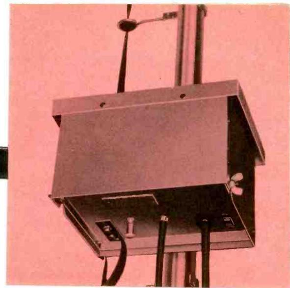
This mast-mounted single-channel amplifier matches a 300-ohm antenna to 75-ohm coax. In addition to providing roughly 16 db gain. Some installations may call for an attenuator or a simple passive matching unit in this spot, while smaller systems may require no unit at all.
