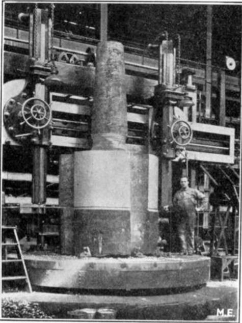
STEEL CASTING FOR ROTOR OF LARGE TURBO-ALTERNATOR BEING MACHINED ON MOTOR DRIVEN BORING MILL.
