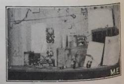
tors, one silicon, the other peroxide of lead, 1 coherer and decoherer (seen on the wall), 1 variable condenser, 1 fixed condenser (not seen in picture), 1 D. P. D. T. switch to receive or to send, batteries to work with the coherer and decoherer decoherer, and 2,000 ohm head set. of these instruments were bought from
