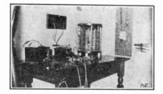
Transmitting, aerial 2 wires, 2 feet apart, 25 feet long, 40 feet high at one end, 30 feet high at the other. Sending helix, glass plate condenser, 1-inch spark coil, spark gap, and key. Receiving, single slide tuner, silicon detector, condenser, and 2 2,000-ohm phones on a headband. With this station I am able to receive 100 to 150 miles and transmit 3 to 6 miles.
