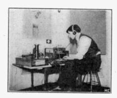
At the right is our sender. In the center of the table is an E. I. Co.'s sending helix, adjustable condenser, key, E. I. Co.'s one inch coil, spark gap, 18 dry cells and D. P. D. T. switch (not seen) in back of the helix to throw in the sending and receiving apparatus.
