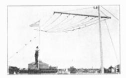
bare copper wires 50 feet long and one foot apart, strung from iron pipe masts on the roof. The iron pipe masts are made of 11/4 inch pipe, supported by guy wires. On each end of my aerial wires I have springs which always keep the wires tight and allow for shrinkage of the ropes in rainy weather.
