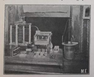
mounted on top of helix, which is E. I. Co.'s; sending condenser is seen to right of helix, which consists of three photograph plates 8x10. Electrolytic interrupter to extreme right was made by myself, large battery jar, lead plate, and copper wire inside of a glass tube; the glass tube has a small hole in the
