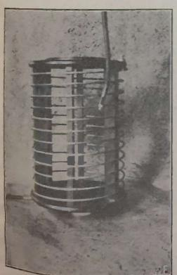
by any student in wireless signaling. The woodwork is of highly finished hard wood which should be well seasoned and dried. The convolutions are of solid aluminum wire and all the metal parts may be readily nickeled and polished,
