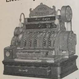
One of the newest features applied to a National Cash Register is a 1-8 horse-power motor. This operates the Register by a mere pressure of the operating key, and stops automatically
