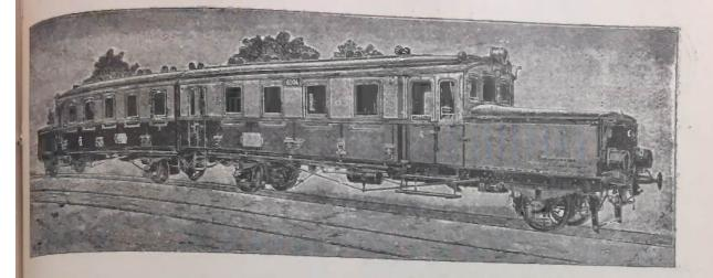
The Prussian Imperial Railroad now has in operation 19 trains of the type shown in accompanying illustration. These trains, composed of two cars, ushally, have in front and in the rear a special tender carrying the storage batteries which are used for the propulsion of the odd looking "train." These trains
