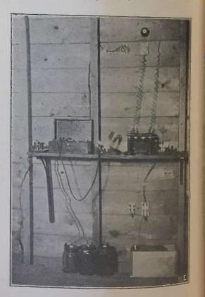
power for the induction coil, and a set of spark balls on hard rubber stands. These stands I made out of the shells from two old telephone receivers, and two binding posts. They can be seen in the picture directly in front of the induction coil.
