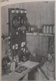
On the front side of the box is a pole changing switch to throw in my where and relay outfit, seen in front of the dynamo. I only use this set for calling purposes, as I find the electrolytic much more sensitive, and capable of receiving messages with greater speed.
