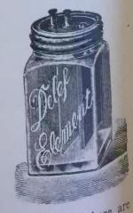
In the small cells there are two ron plates and one zinc plate on open circuit 0.9, closed circuit volts. volts. Capacity of smallest cell made
