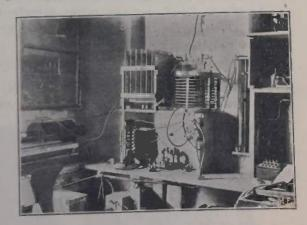
The tuning coil is shown at the right of the picture. It is made in two sections, 23 D. C. C. wire, with two sliding contacts. The connections are such that all wire in both sections above the top sliding contact is in series with the aerial, while the lower sliding contact grounds the tuning coil. I find this coil gives very good results, besides being very compact.
