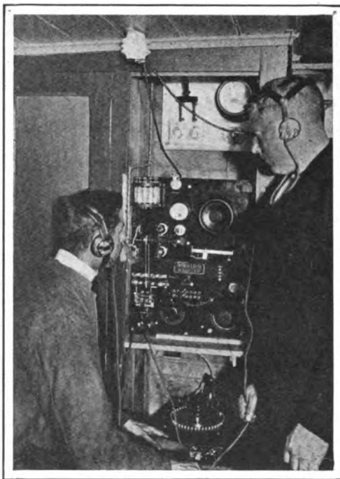
THE ONE-HALF KW. STATION ON BOARD THE "DROSSEL," SHOWING THE SEPARATE RECEIVING AND SENDING OUTFITS
