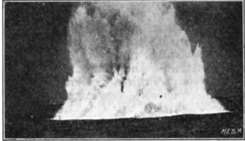
BLASTING IN THE DETROIT RIVER
