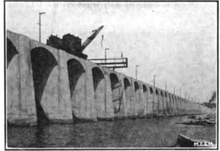
A SECTION OF THE DAM SHOWING SPILLWAYS
