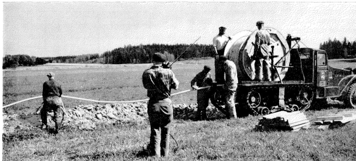
Figure 7—Rear view of vehicle showing mounting of cable reel and method of paying out cable into trench.
