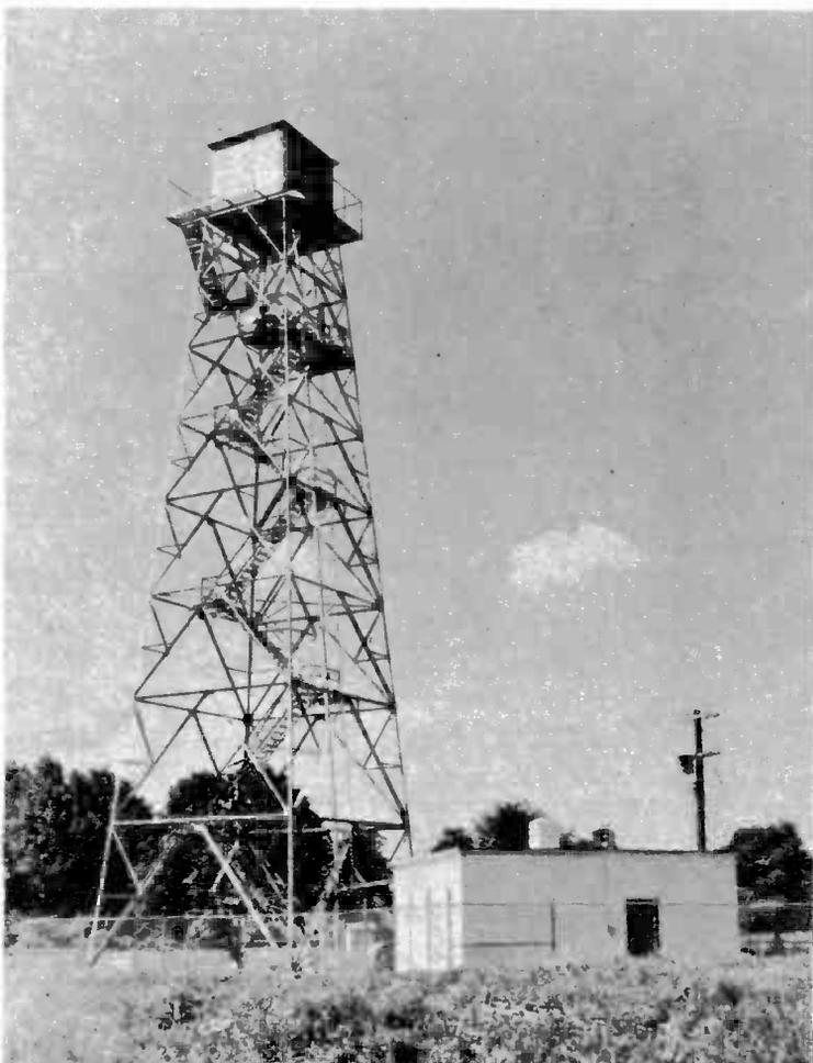
At left is one of the many microwave towers that provide Western Union communications between New York, Philadelphia, Washington, and Pittsburgh. At second level (from top) is "dish-pan" antenna that beams waves, much as a searchlight does. Other antennas are in the enclosure.
