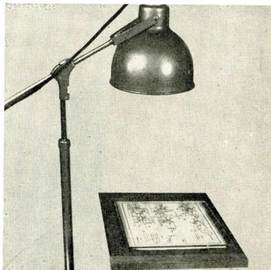
**Sun lamp** provides illumination in this set-up. Drawing lies on top of sensitized paper.
