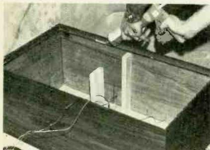
Glue around edge of cabinet, don't leave any gaps. Wire up the midrange enclosure.
