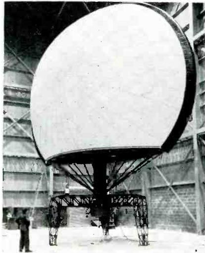
**COLLAPSIBLE** magnesium base aids mobility of this new portable paraboloon radar antenna with an inflatable reflector, developed by Westinghouse for the Air Force as . . .
