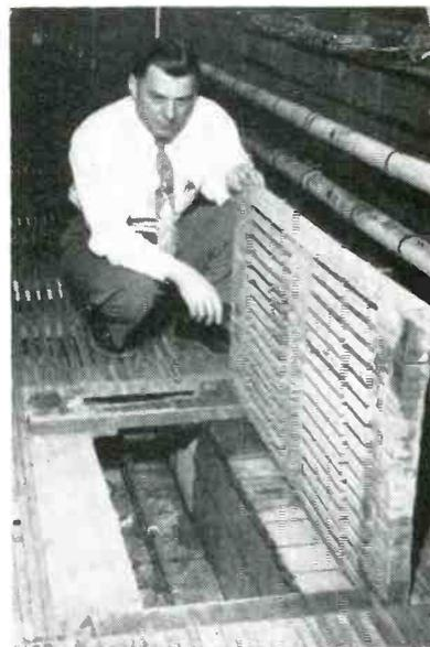
Acid-proof brick trench 15 inches deep carries away corrosive acids in plating room of tube plant
