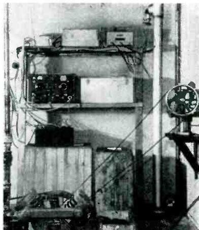
Interior installation at Holland Rock. On top shelf, from left to right, are: radiotelephone-transmitter control; time-sequence control; microwave receiver. Radiotelephone transmitter and batteries for receiver are below. Air compressor at lower left drives foghorn coding timer at right
