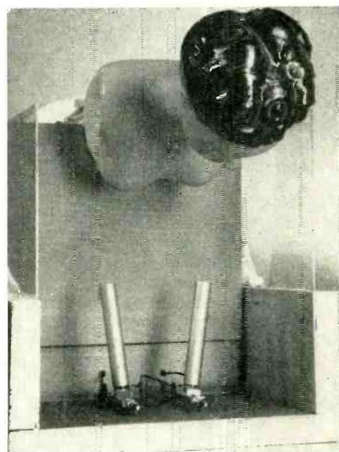
Model of one method for systematically scanning the breasts, suitable for mass surveys. Motor reciprocates transducers at the bottom of a large water-filled tank
