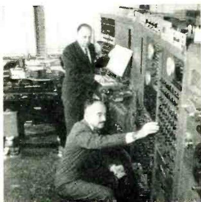
EXPERIMENTAL electronic instrument to synthesize familiar sounds and to create an unlimited range of tone variations and rhythms, developed and recently demonstrated by RCA, is operated by H. F. Olsen, rear, and Herbert Belar of the firm's research center in Princeton, New Jersey.
