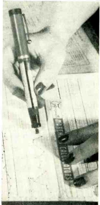
Method of using sliding-average computer. Straightedge is held on zero line of chart to serve as convenient stop
