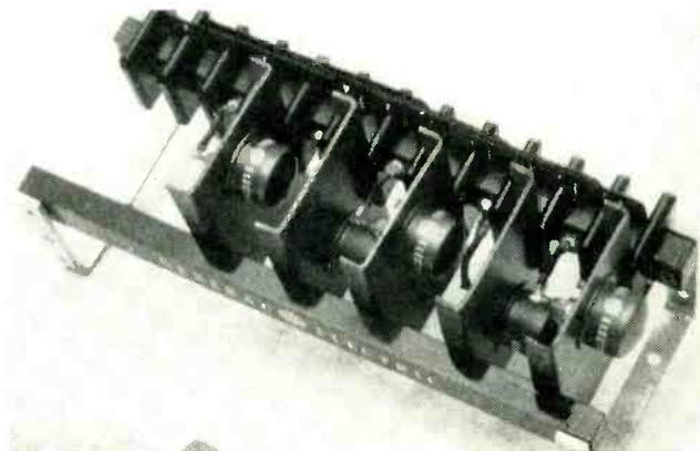
FIG. 8—Stacked germanium rectifiers, under development, provide 5 amp d-c output per cell
