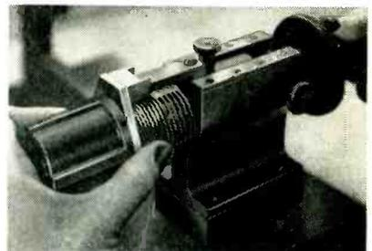
Holding housing against gate while turning crank to thread coil and drum into housing
