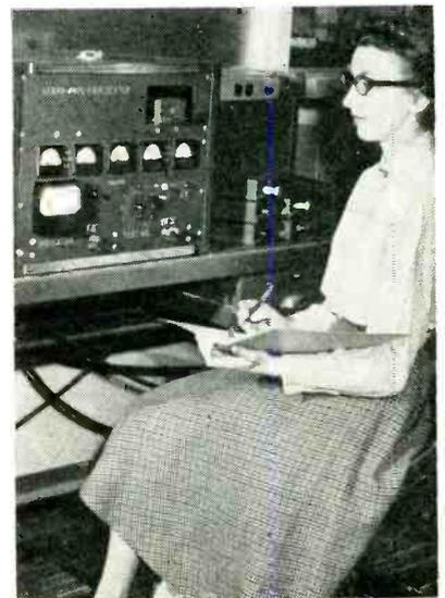
Production-bench setup for testing packaged servo amplifiers
