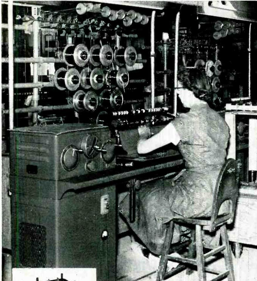
At the Freed Transformer Company, well known manufacturers of electronics components, Leeson No. 108 Hand-Feed Coil Winders have replaced obsolete winding equipment. Here's what the president of Freed reports about the new installation:
