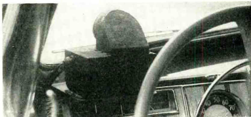
Method of mounting dimmer in automobile for tests. Unit here is made more compact by mounting scanning disk horizontally and using mirror to bend light beam
