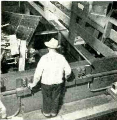
In the Weyerhaeuser Timber Co. sawmill at Longview, Wash., mill ends and edgings are recovered for production of pulp. The salvage is conveyed to chipper machines that cut the scrap into small pieces before being sent on to a chemical digester.
