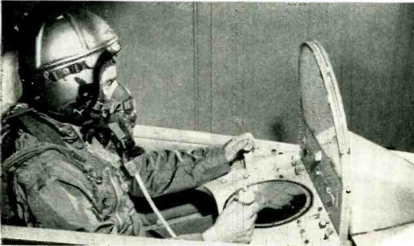
Naval aircraft may soon use a transparent television-type tube as combined inner windshield and radar display. In addition, other information could be similarly displayed before the pilot by means of another flat cathode-ray tube set into a shallow instrument panel. The tube has been developed by the West Coast Electronics Division of Willys Motors. It may have future use in home television receivers.
