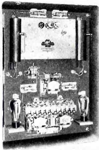
from a-c power have been announced. One model is a general purpose, reversing type applied to a 2 hp, 230 volt d-c motor, and the second is a special control for an abrasive surface grinder. For any speed setting, performance is practically equal to that of a synchronous motor even with a suddenly applied load.
