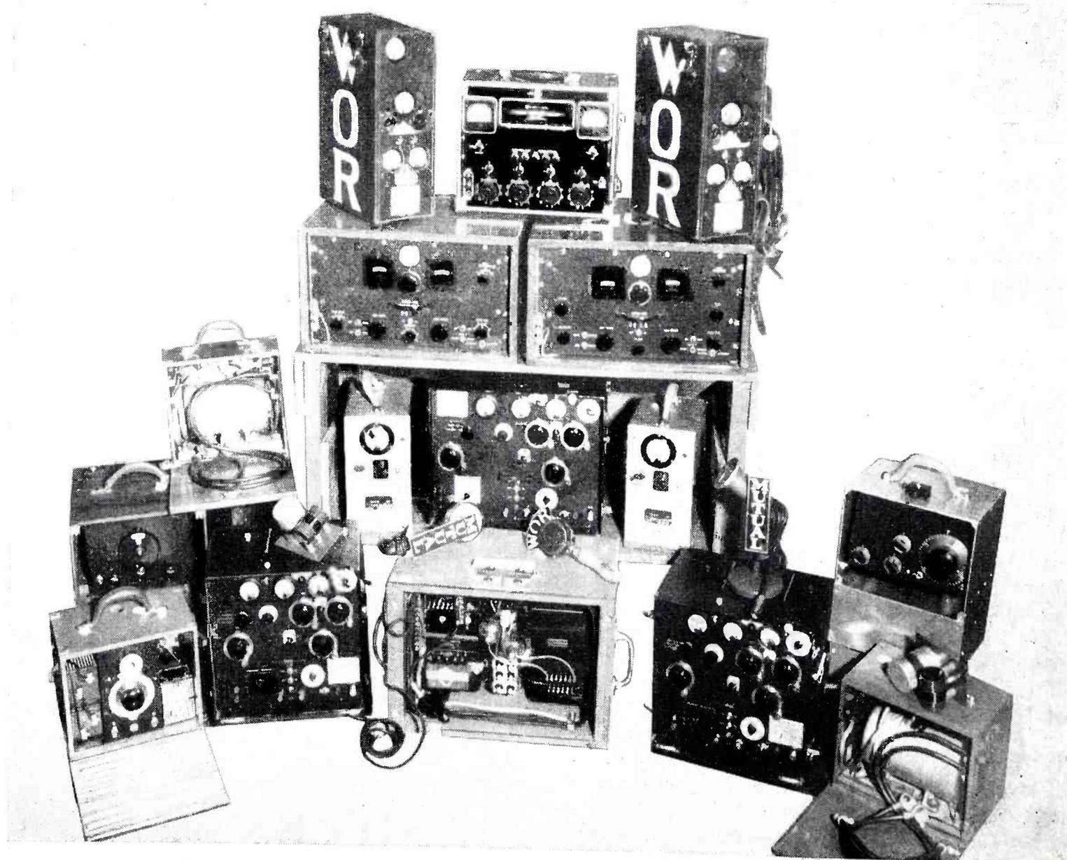
Part of short-wave field equipment for broadcasts from locations without wire lines
