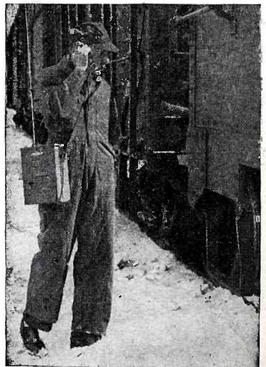
Track-side railroad crewman communicates with conductor over two-way handie-talkie developed by Bendix engineers
