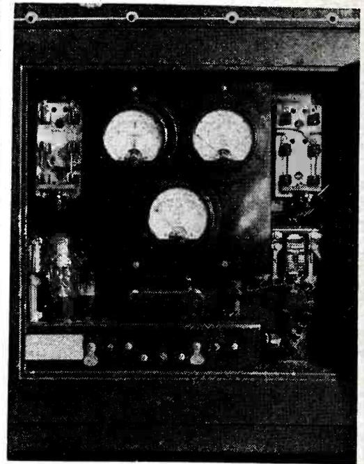
A constant d-c supply to a rotary converter from the unit above provides a stable a-c voltage for critical equipment
