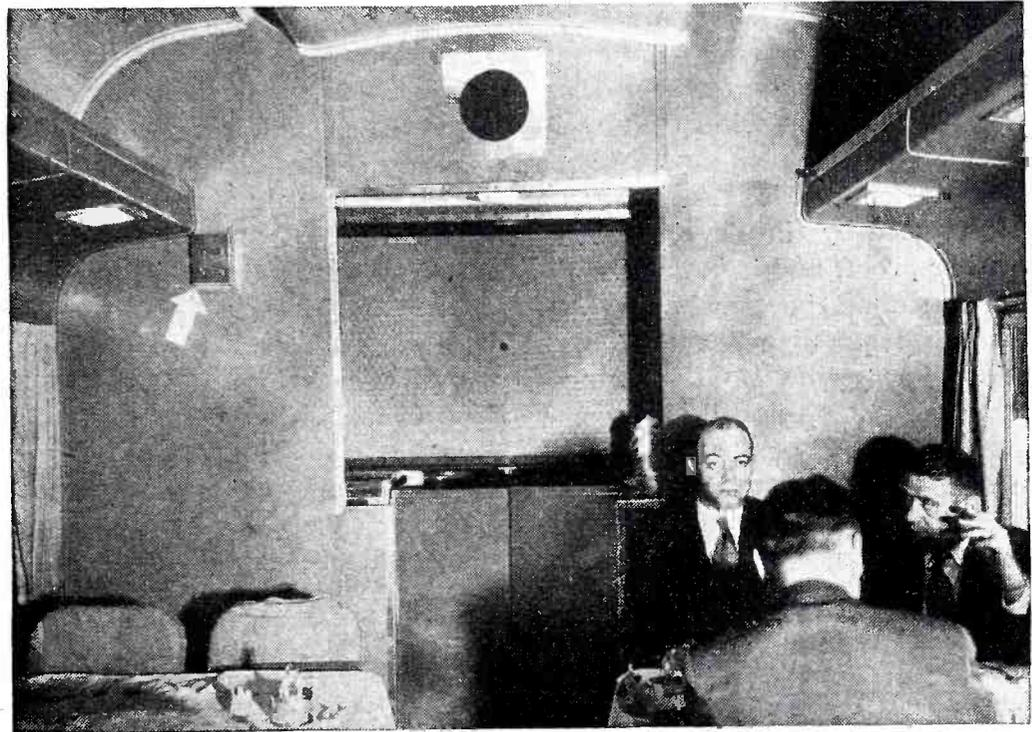
Remote control (arrow) and loudspeaker near ceiling in a Rock Island dining car
