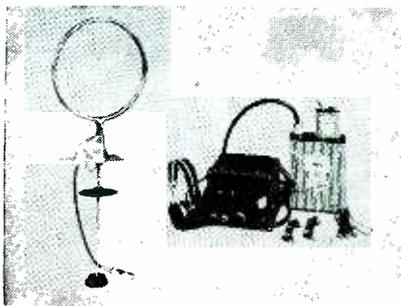
receiver tunes aircraft range beacons in the frequencies 195 to 405 kilocycles. The equipment is simple to install, weighs 12½ pounds, and sells for \$159.50.
