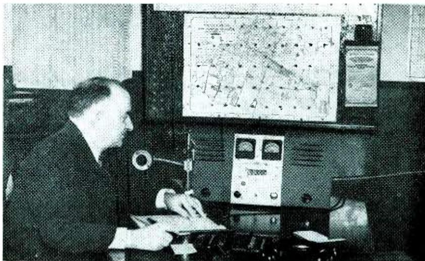
Dispatchers' desk showing dual telephone positions for incoming calls, radio microphone, and remote control unit that is operated by foot switch
