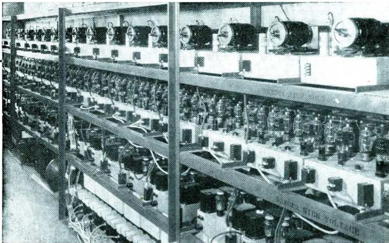
Equipment for the production testing of aircraft tachometers. Pole wheels are on the floor, in the background, with frequency-selector relays and stepping switches in the foreground. Powerpacks are on the first shelf, two-phase amplifiers on the second and synchronous motors driving tachometer generators on the third
