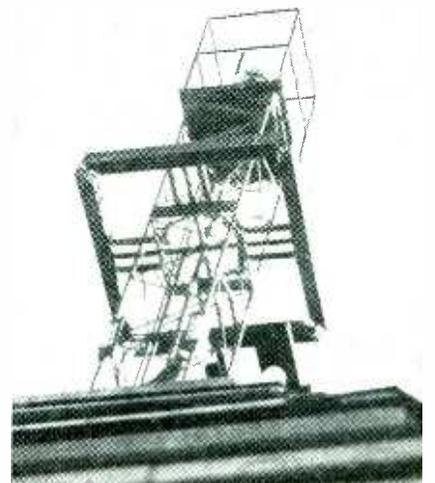
First square-loop section of the antenna as it cleared the roof
