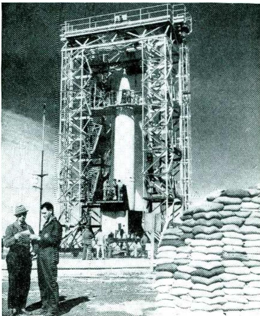
Gyro steering control and telemetry of 28 instruments in flight is done with G-E equipment in tests of the V-2 rockets. The gantry crane shown above has expedited preparation and assembly of the electronic control gear in the missile
