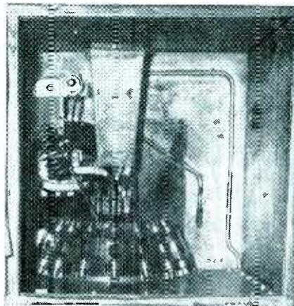
Grounded-grid oscillator using water-cooled 9C21, the leads of which can be seen projecting above ring of vacuum capacitors that ground the grid, dissipates 50 kw at plate. Rectifier in grid circuit, not shown, stops damaging grid emission
