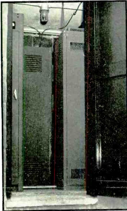
**REPEATER BUILDING INTERIOR**—This typical hilltop structure contains a 50-watt, 116-119 Mc amplitude modulated repeater transmitter, a 250-watt, 33.94 Mc frequency modulated transmitter and a steel-enclosed rack and panel unit housing control receivers and automatic relays
