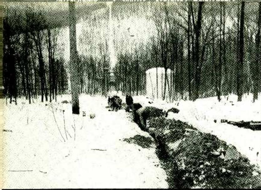
**IN THE TRENCHES**—Over six miles of cable carrying power and remote control currents was laid in 18-inch deep trenches dug in the dead of winter. In the background is a tunnel portal and, rising above it, a cut through the wooded hillside up to a mountain-top repeater station
