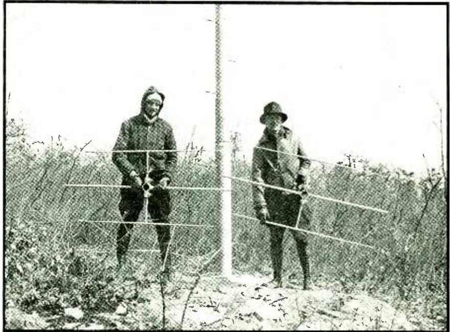
**READY FOR A CLIMB**—Two uni-directional arrays of the parasitically excited director and reflector variety, on the ground at the base of a concrete-embedded repeater station pole
