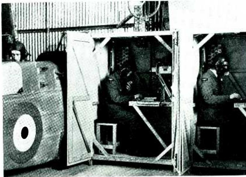
The R.A.F. trains operators under conditions simulating those which they will later encounter in flight. Here are three operators receiving or giving instructions in code transmission and reception in order to qualify each as a wireless operator gunner
