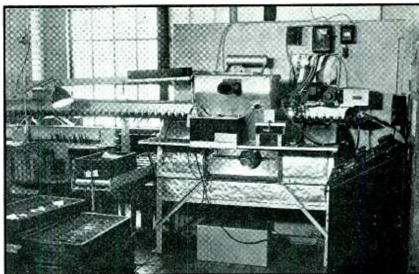
Equipment used to test an interior lead soldered joint in table knives by means of x-ray gas ionization. The x-ray tube is shown beneath the bench and the knives to be tested pass through an opening to a ionization chamber. The amount of lead in the joint determines the degree of ionization of the air in the chamber
