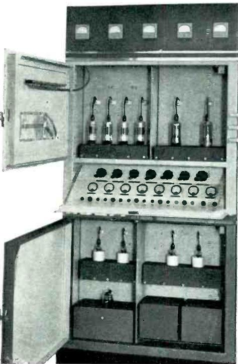
★ **MODULATOR CUBICLE**—Lower door opens to make it easy to check relay operation.
