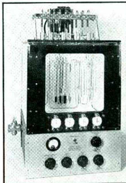
Fig. 3—The constant temperature bath mounted atop the regulator. The four knobs at the bottom control the temperature setting
