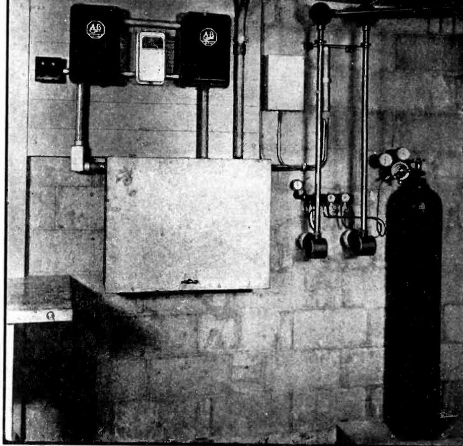
Fig. 7—A neat gas-filling installation, at WKBN. Note that a duplicate cable is maintained as a spare (Communications Products)
