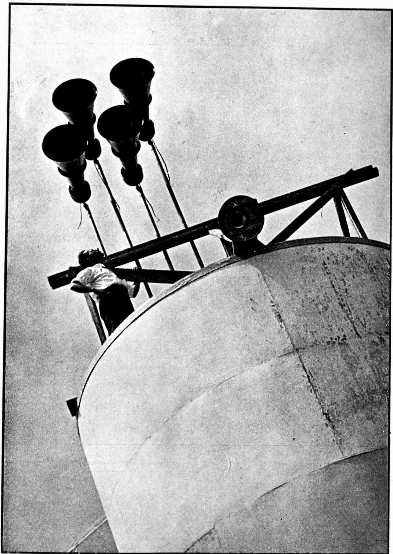
**Sound . . .** Experimental 100-watt loud speakers on test during early days of New York World's Fair construction. In spite of steam shovels and other noise making machinery, the battery covered an area of  $\frac{1}{2}$  mile radius
