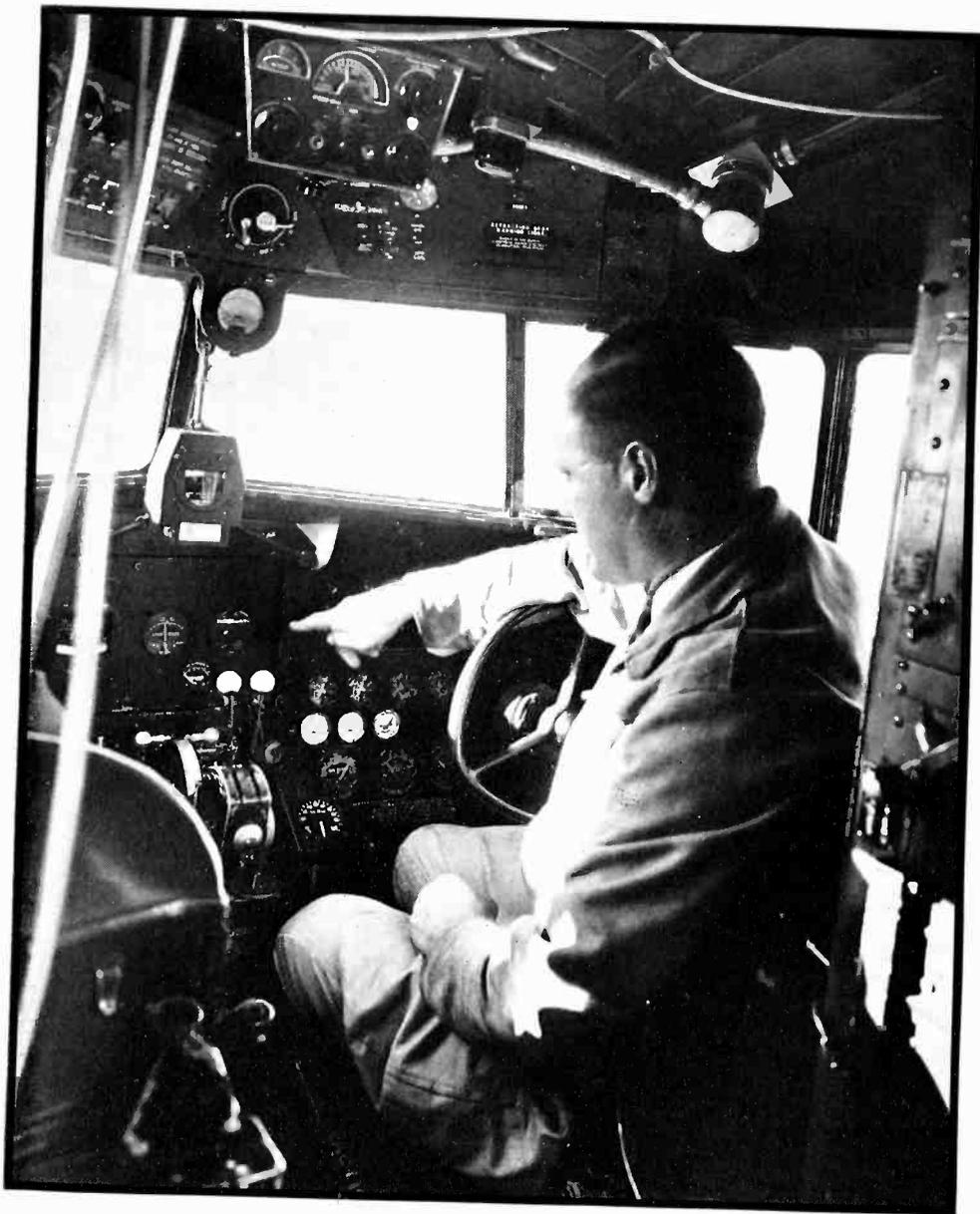
*The pilot's position in a TWA Douglas Transport, shown to the right. The compass indicator to which the pilot is pointing is only one of 25 dials and gages he must watch.*
