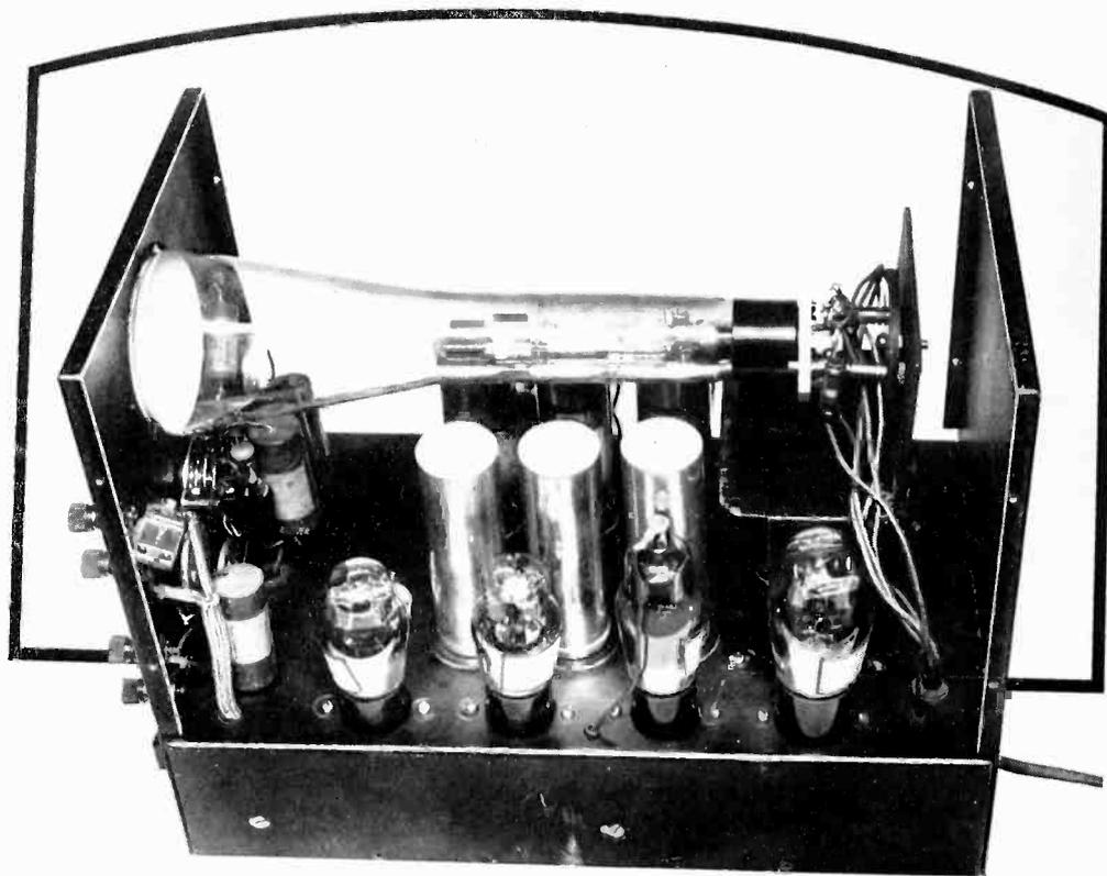
*Cathode-ray resonance curve indicator using capacity control tube as part of sweep circuit*
