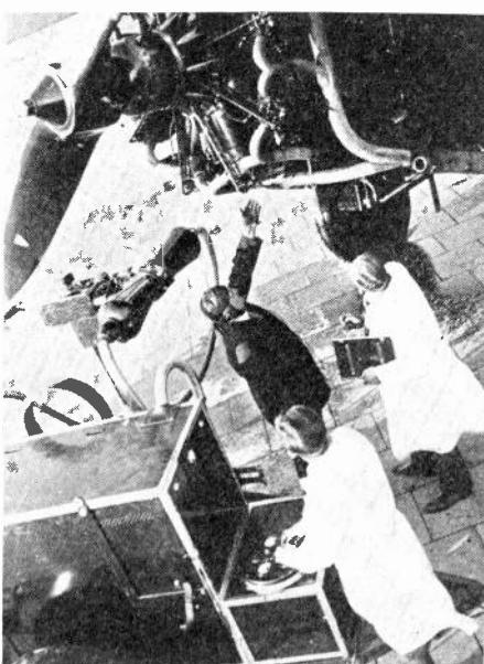
At the Fuhlsbuttel aerodrome near Hamburg, Germany, a portable X-ray outfit can be wheeled out onto the field and used to inspect propellers, engine parts, and gear, detecting flaws invisible to the eye.
