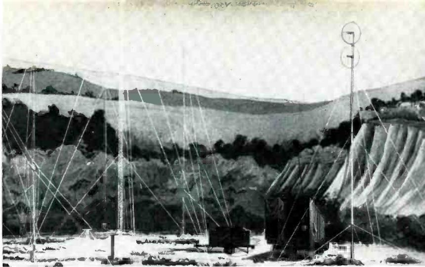
Artist's version of a field setup of the system. One of the two vans and power trailers is shown along with antennas for the u.h.f. relay link (right) and the rhombic transmitting and double-doublet receiving antennas (left). The rhombic's height has been exaggerated and its size reduced in this photo.
