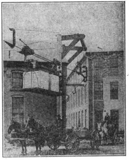
Telpher in use at the Arnold Print Works, North Adams, Mass. It operates among the various buildings, hoisting the load from the road or wagon and carrying it down the alleys and into the various floors of the building.
