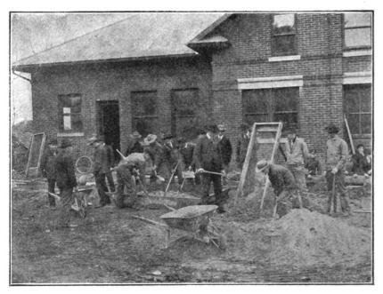
Fig. 1. Method of Screening Sand from Gravel
