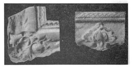
Fig. 3. Plaster Molds of Details
