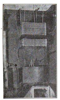
Fig. 6 Transmitting Inductance and Oil Condensers
