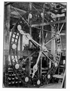
Fig. 7 Showing construction of dial of clock on Federal Building, Newbern, N.C.
