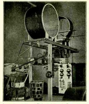
Fig. 6. The 100 Kilowatt, Undamped Wave, Arc Transmitter at Arlington (extreme left) and Huge Tuning Inductances for It.
