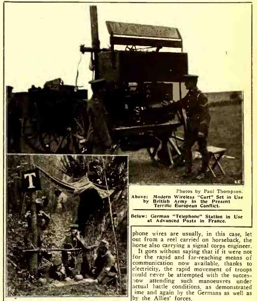
Our first photograph shows a modern wireless "cart" set as used in the British army. These sets are very compact and can be unpacked and set up, ready for operation in transmitting radiograms over sections of several hundred miles, in a few minutes' time.
