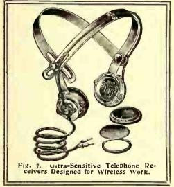
On the permanent magnet 4 is mounted a pair (sometimes only one) of soft iron pole pieces on which are wound many turns of fine insulated copper magnet wire. For all regular telephone work the coils have a total resistance of 75 to 80 ohms. Wireless receivers have from 1,000 to 3,000 ohms resistance each usually, as the current used is very minute, or a few millionths of an ampere.
