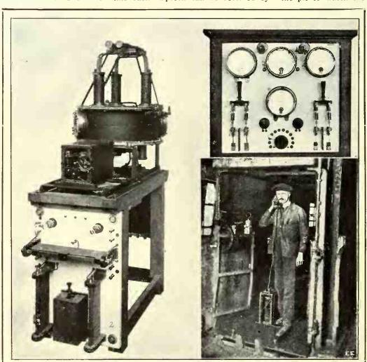
At Left, New French, "Colin-Jeance" Wireless Telephone Apparatus. Top (Right) Switchboard For This Set. Below (Right) New Type of Mine Wireless. Telephone Devised by Herr Reineke, of Germany.
