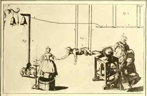
Fig. 2. Experiments with the Early Static Electric Generators Were Mostly Carried Out With a "Human" Prime Conductor as Here Shown.
