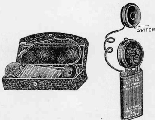
Fig. 1. The "Electro" Detectiphone aiding partially deaf people, and with ordinary usage, say of
