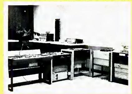
A look at part of the room. Included are a mixing desk, ¼-inch recorders, a turntable, and a new 8-channel recorder.
