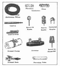
FIG. 2. A few of the common parts required for antenna systems
