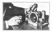
Removing a tube shield for tube inspection
