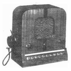
Courtesy Operadio Mfg. Co., St. Charles, Ill. Station unit of the Operadio type C intercommunicating system. Each station uses the same master unit, and can therefore call any other station at will. Up to eleven stations may be used in a system. Each unit has a combination on-off switch and volume control, a "listen-talk" switch, an earphone with switch for privacy, a jeweled pilot lamp, and ten station-selecting switches.
