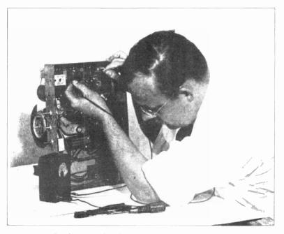
Service man checking chassis with an ohmmeter
