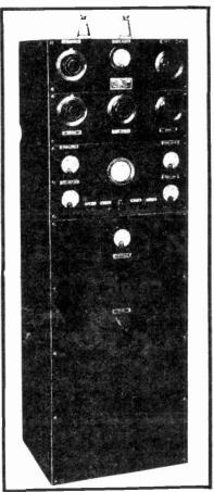
FIG.1 A 100-Watt Transmitter.
