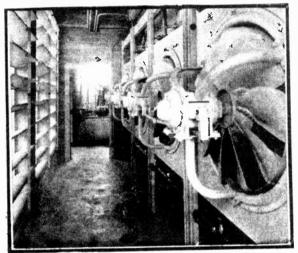
FIG.12 Cooling Fans and Radiator System.
