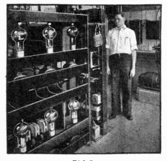
FIG.I Bank of Rectifier Tubes In a Short-Wave Broadcast Station.
