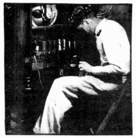
FIG. 1 Checking a Receiver With an Analyzer.
