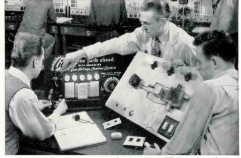
Here you see an instructor giving a demonstration on different makes of low voltage house wiring control systems. These controls are being used more and more in modern buildings.
