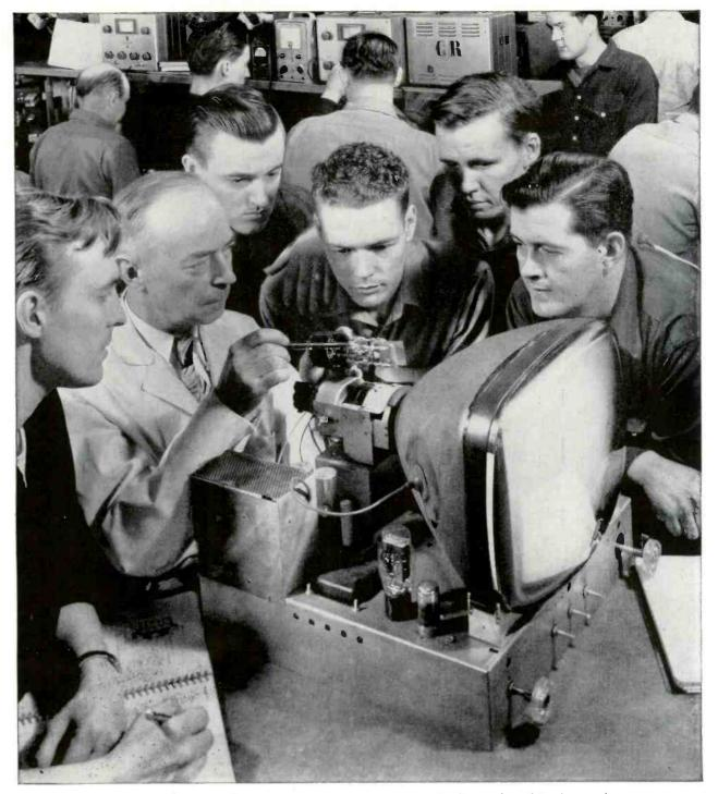
In the above phota we show an instructor giving a demonstration and explanation on how basic principles are utilized in the electron gun of a Television Picture Tube. The electron gun is the heart of a Cathode Ray Tube used in Television.
