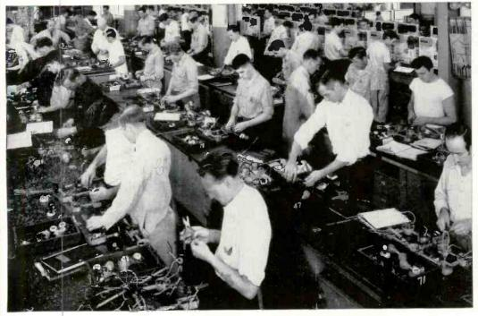
General view of a section of Basic Electricity and Circuits. Notice the large and well lighted shop. The men are wiring and testing light control circuits in their first small conduit loyout, and getting real practical experience in the handling of tools and the use of various kinds of switches.
