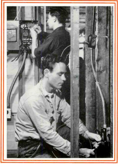
Another important part of house wiring is pulling the wires through the tubing after it has been installed. Here you see students getting practīcal experience on wire pulling.
