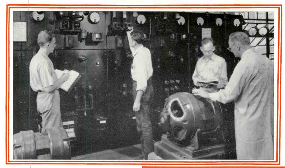
Here are students getting real operating experience on a large power D. C. Switchboard. They are taught to connect and operate gemerators in parallel, and to take care of circuit breakers, switches and instruments. This kind of training is valuable in power plant or substation operating work, and many of our graduates have good jobs doing this work.
