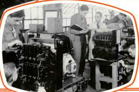
The students above are getting actual operating practice on a large A. C. Switchboard. Here they are taught the operation and care of meters, circuit breakers and switches, and how to synchronize and operate alternators in parallel.
