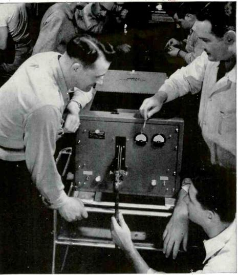
The unit shown above is a commercial High Frequency Induction Heater of the type that is used for soldering and heat treatment of metals.
