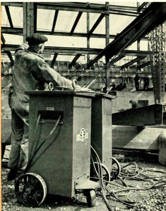
An early 300-ampere a-c welder (left) on a construction job. The modern "65-line" family, so called because of the low open-circuit voltage, is built in ratings of 200, 300, 400, and 500 amperes (below) and 600 amperes (above) output.
