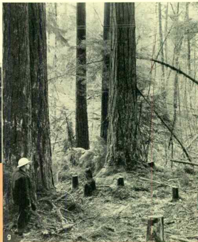
Plywood (e), with greatly improved glues and new curing techniques, contributes much to better utilization of some woods. At (f) is shown salvage logging using equipments designed for that job, while (g) illustrates prelogging of small trees to prevent their destruction when big ones are felled.
