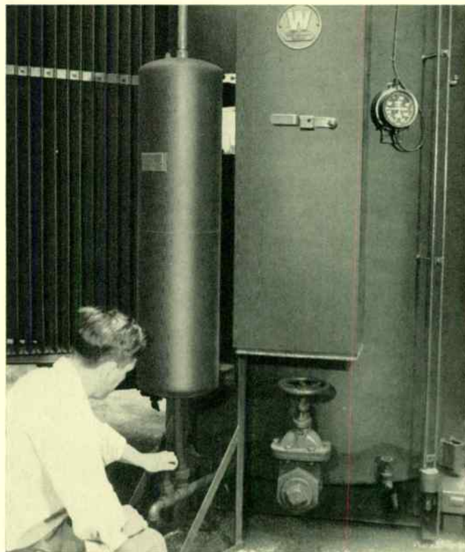
The magnetic temperature indicator (extreme left) is reset by an external magnet. At left is the liquid-level indicator. The oil conditioner (below) maintains the qualities of transformer liquids.
