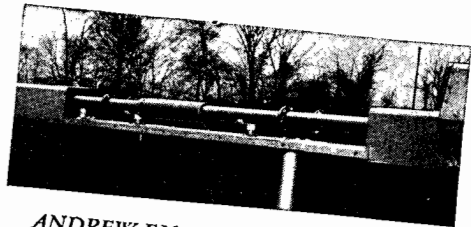
ANDREW FM-AM isolation section with cover removed, revealing two 3/8" FM transmission lines and expansion joints.
