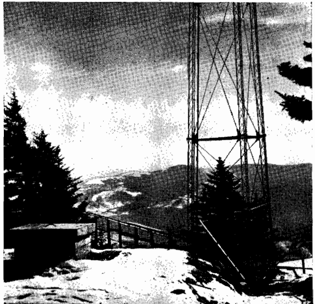
Atop White Top Mountain where the WOPI-FM antenna and transmitter were installed. At right is the antenna tower base and at left the 11,000 gallon reservoir.
