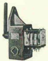
Fig. 42—2-Pole Auxiliary Switch.
