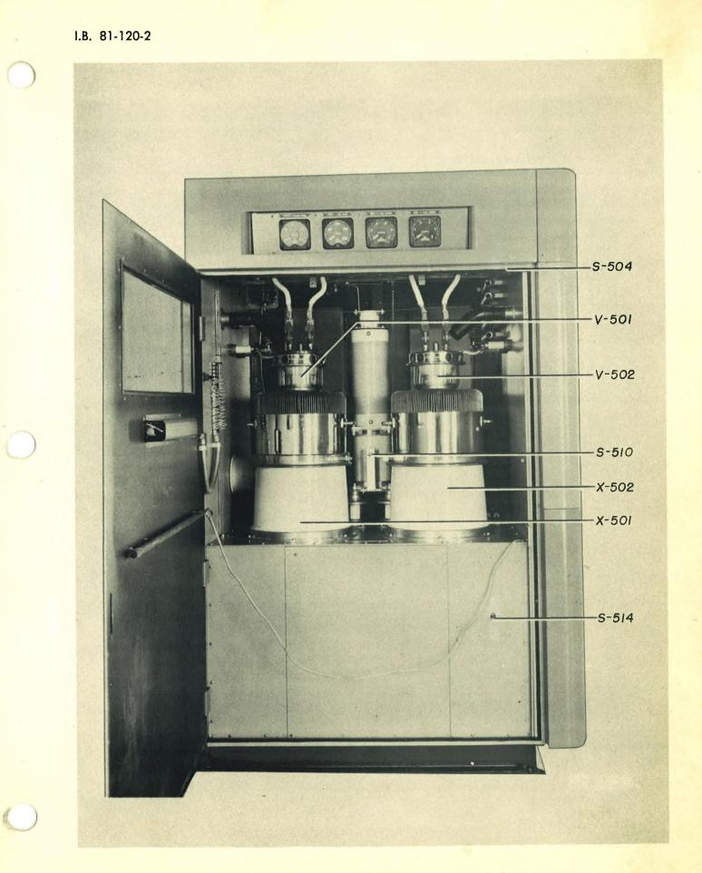
FIG. 24. Right Power Amplifier Cubicle, Interior, Front View (Photo C-12140)
