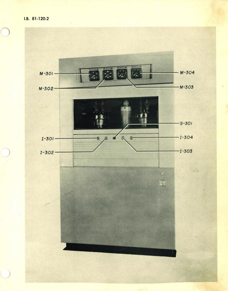
FIG. 16. Left Power Amplifier Cubicle, Front View (Photo C-12128)
