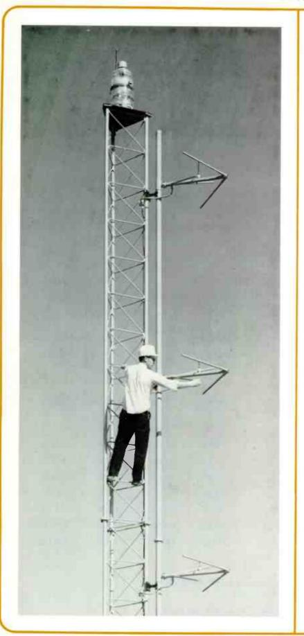
The best state of the art FM transmitting antenna, the JAMPRO CP produces circular polarization by a patented Jampro method.
