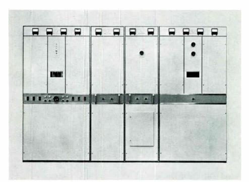
type 8 FZ 510 broadcast transmitter comprising from left to right: power supply, modulator, driver and output stage
