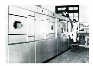
installing a Philips 50 kW short-wave broadcast transmitter at Radio Goa Broadcasting Centre
