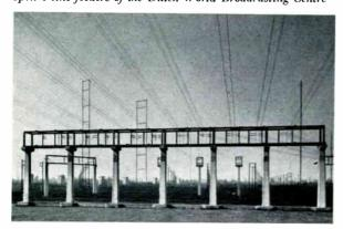
The ever-changing propagation conditions often necessitate the use of two different aerials for broadcasting in one and the same direction.
